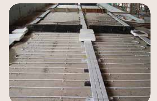
Close up view of the PEX pipes installation in Floor Slabs
