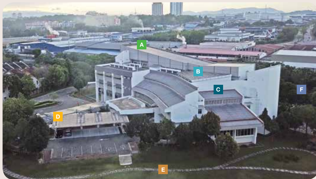
MGTC's GEO Building
